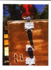
View of the pump controls at the lift station. Pump #2 was in automatic mode, and Pump #1 was off at the time of inspection. An alarm light was present, but was not lit.
