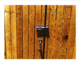
View of the access gate at the lift station. The gate is not locked and is only secured by a slide bolt.
