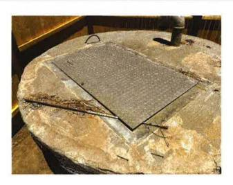
View of the vault at the lift station. A piece of rebar was wedged under the hatch for ease of opening.
