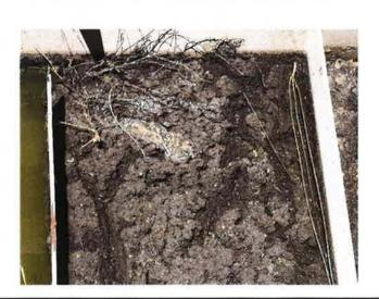
View of the sludge layer that is present in the chlorine contact basin.
