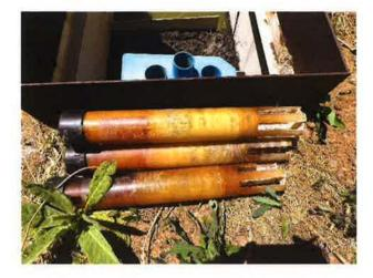
View of the chlorine tablet feeders that are lying on the ground outside of the unit.
