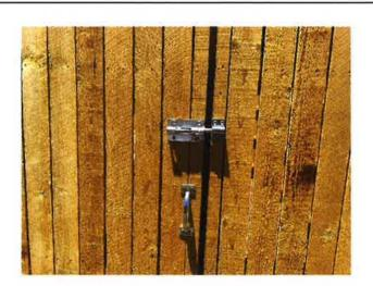
View of the access gate at the lift station. The gate is not locked and is only secured by a slide bolt.
