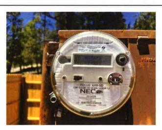
View of the meter at the lift station. A pump was audibly heard to be running, although the meter was reading zero at the time the photo was taken.
