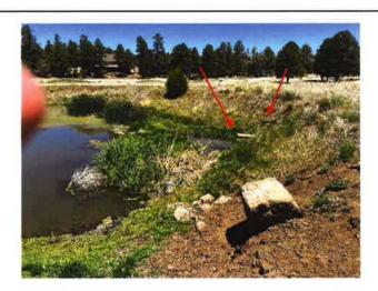
Alternate view of the northeast end of the effluent pond. Discharge pipes are visible; one appears to be effluent, and the other may be storm drainage.
